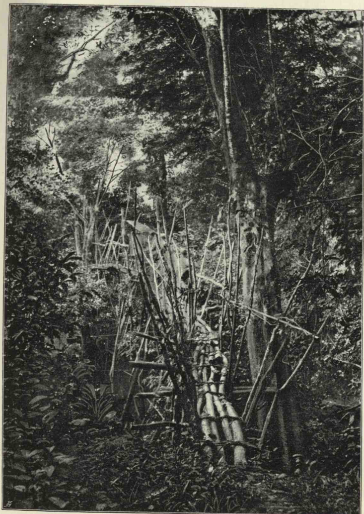
Fig. 6.—A HIGH TRESTLE BRIDGE OVER DEEP RUNNING STREAM. SHERBRO DISTRICT.
