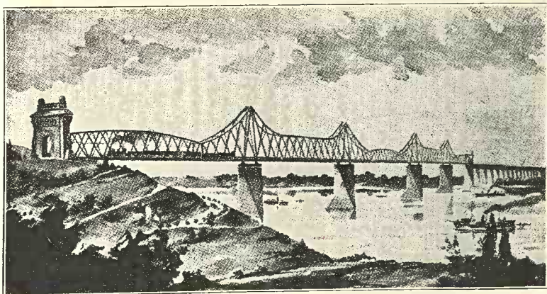
BRIDGE OVER DANUBE RIVER AT CERNA VODA, ROUMANIA, DESTROYED BY THE GERMAN ARMY
