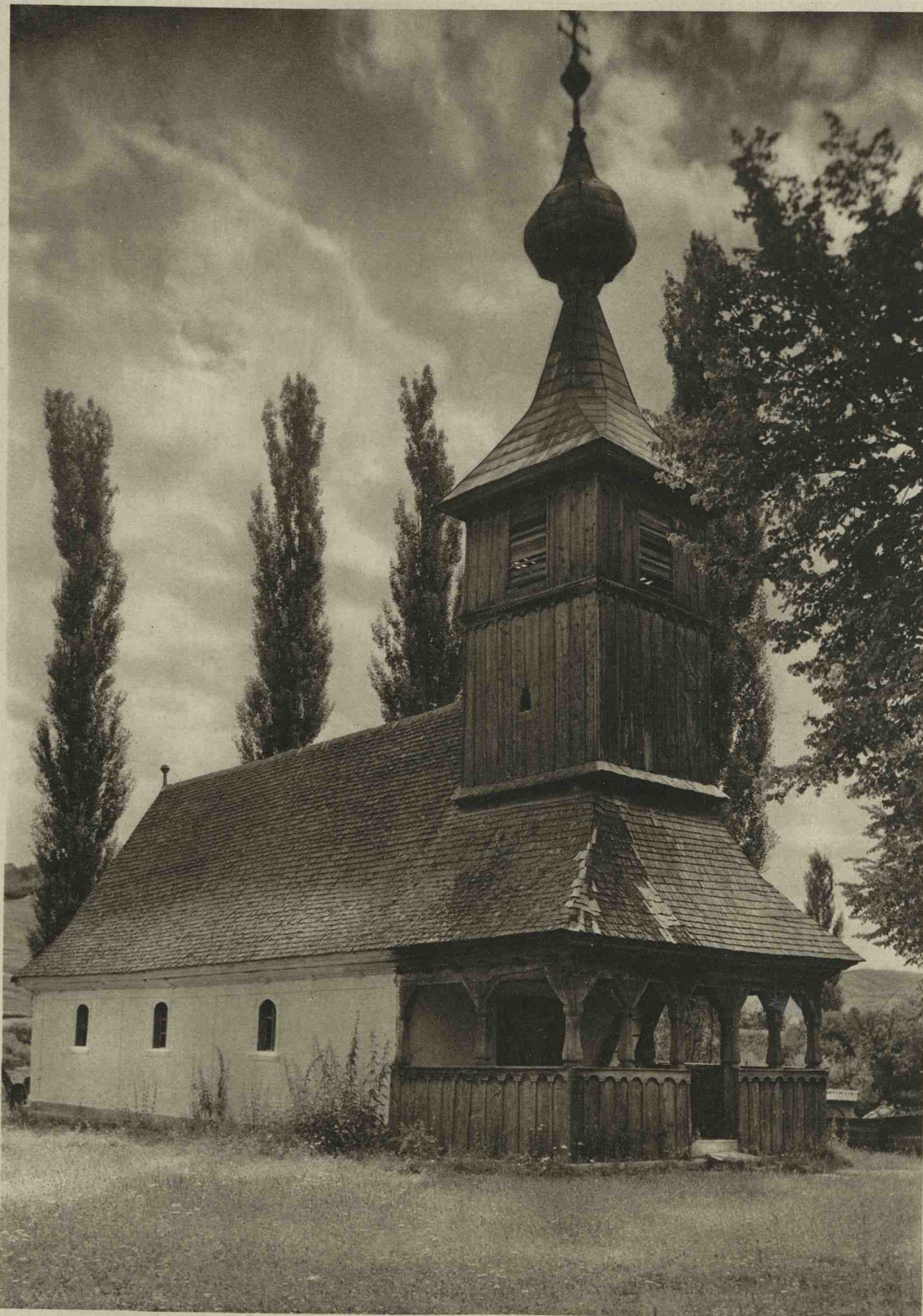
Holzkirche Wooden Church
