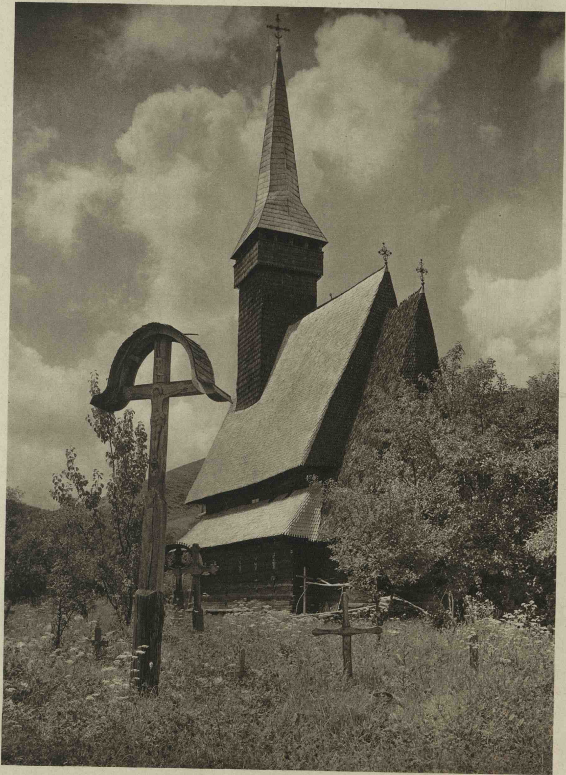
Holzkirche Wooden Church
