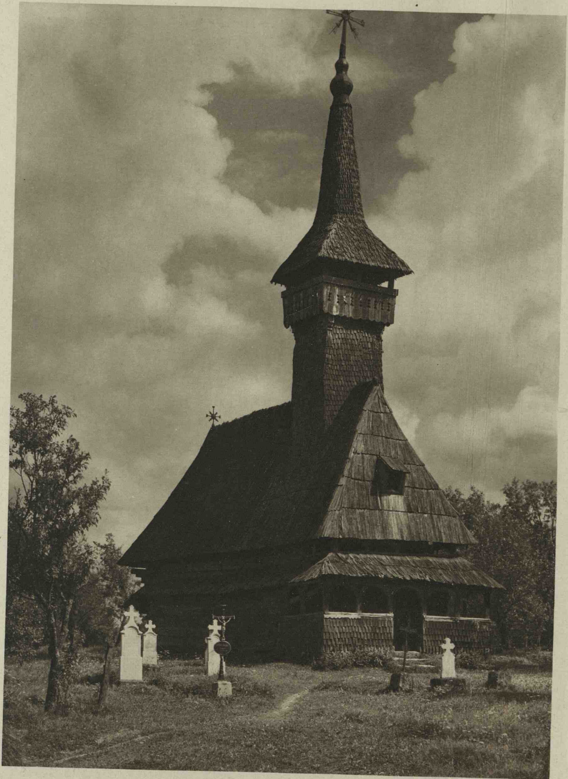
Holzkirche Wooden Church
