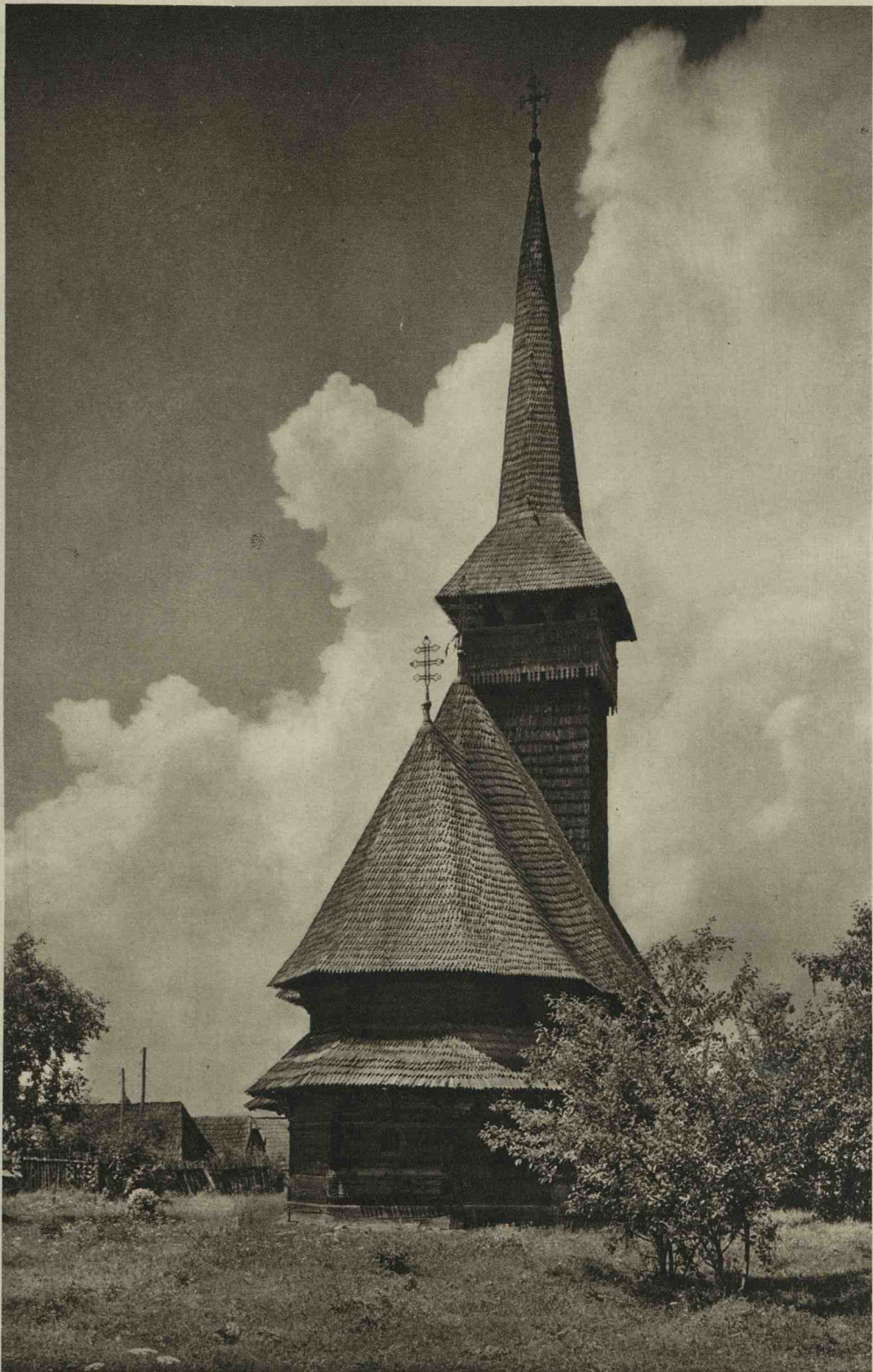
Holzkirche Wooden Church
