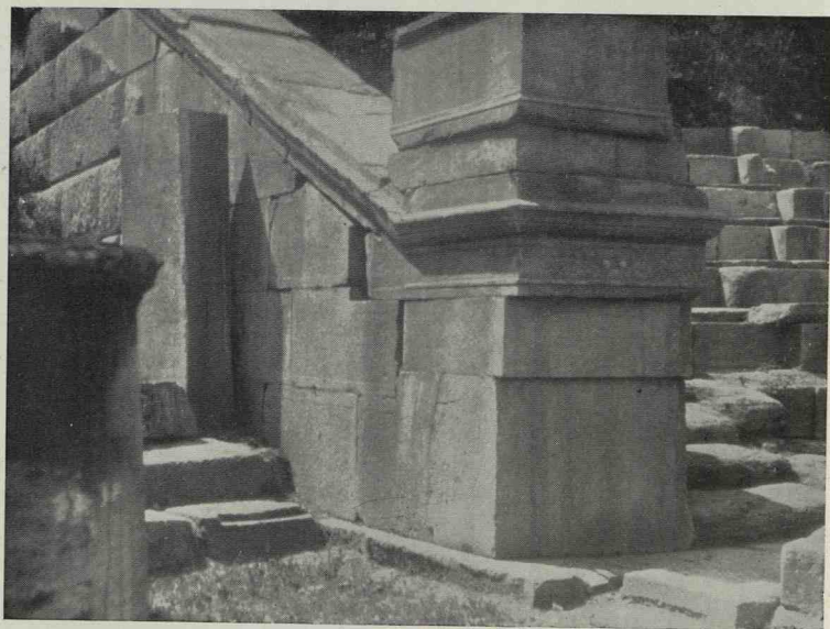
(b) The same. Die-wall at end of seating.
