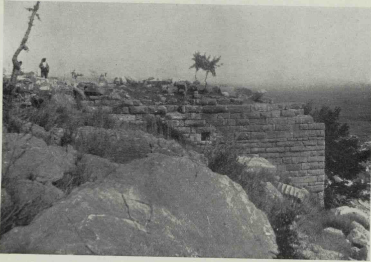
(a) Priene. Bastion forming platform of Athena temple, from west.
